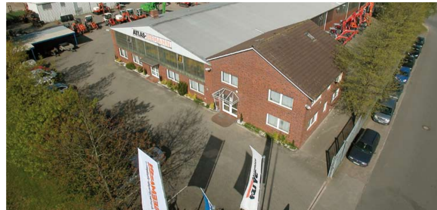
The business premises of our longtime contractual partner Seemann
